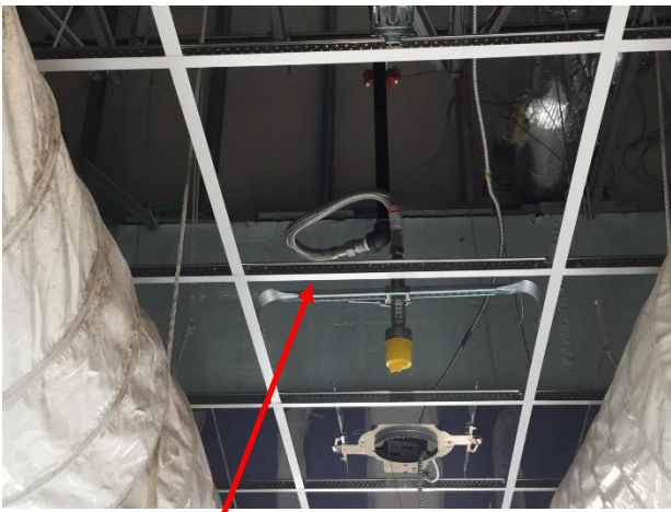
Failing to maintain the 4" minimum radius & number of bends allowed for 2' hose in violation of the U. L. Listing
