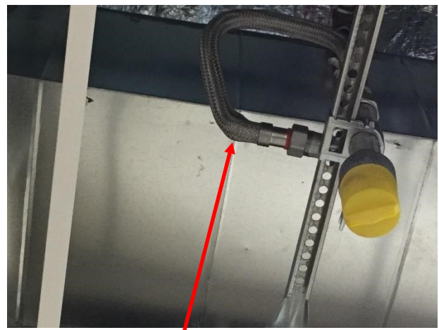
Crimped the hose during installation to achieve center tile
